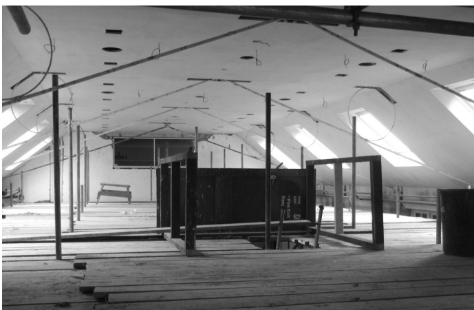
View from the scaffold— ceiling works at the Victory Hall
